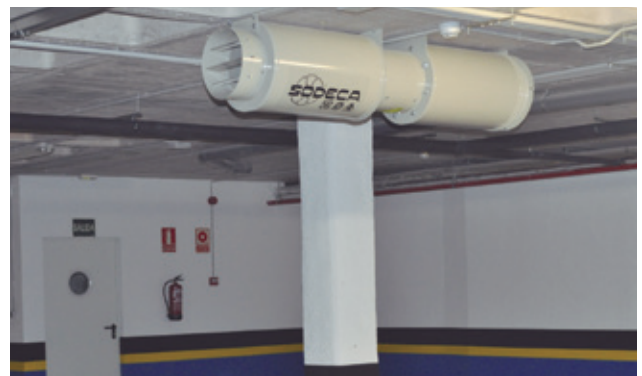
THT/IMP instalado en parking
